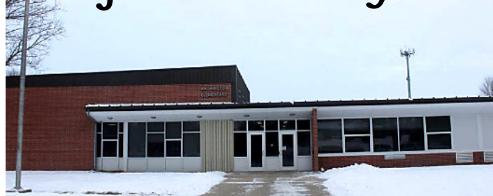
2005 - 09 WASHINGTON ELEMENTARY 500 E. 14TH ST.
